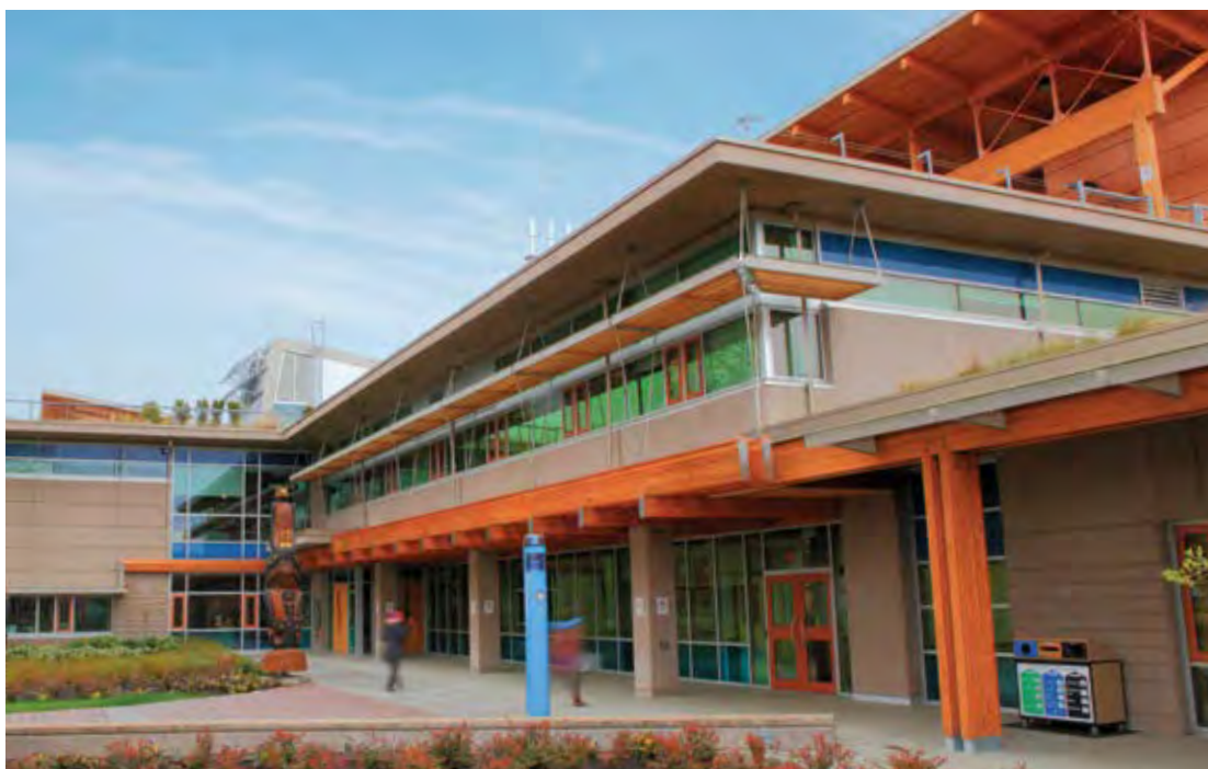
Vancouver Island University, Cowichan Campus Source: Vancouver Island University
